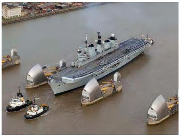
Constructed between 1974 and 1982. the Thames Barrier is the world's largest navigable flood barrier and some consider it to be the eighth wonder of the world. A flood defence barrier was considered to be imperative because high water levels at London Bridge have risen by almost a metre per century, due to global warming and the embanking of the river.
